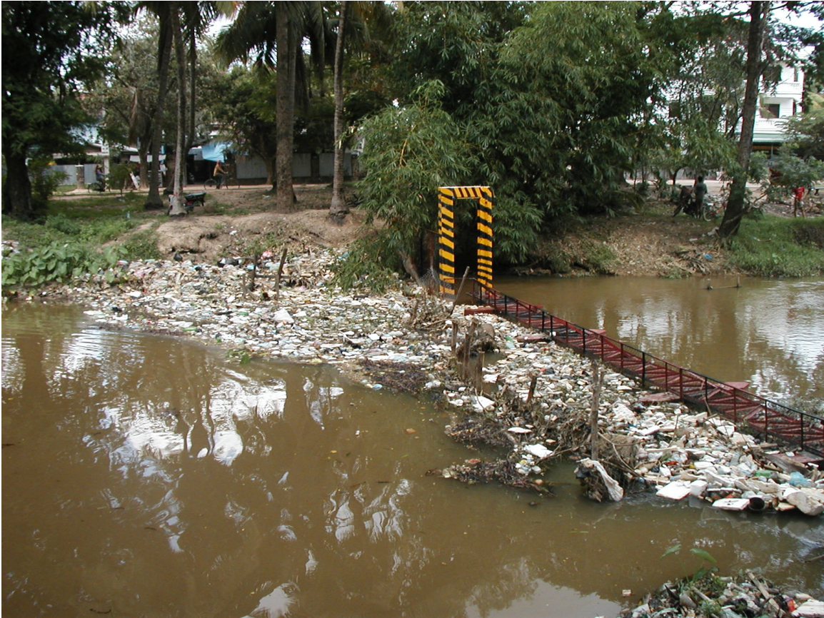
Figure 2. Barrier to waste across the Siem Reap River upstream of the Town of Siem Reap
