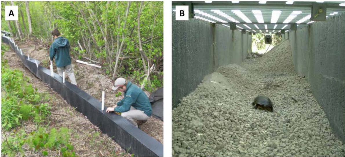
Figure: An example of conservation infrastructure for freshwater turtles called an ecopassage. Photo A is the implementation of the short fence parallel to a road that used to guide animals towards the tunnel for safe crossing. Photo B is the ecopassage tunnel under a road.
